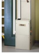
Upgrading to a two-stage, variable-speed gas furnace can be beneficial in the summer. Your outdoor air conditioner or heat pump uses the furnace blower to distribute air throughout the home. The variable-speed feature helps reduce humidity levels inside the home and helps run the system more efficiently during the cooling season.
